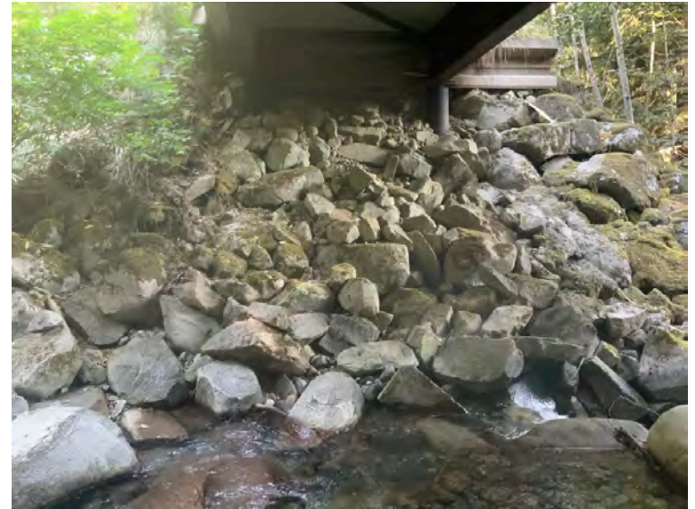
Left Bank Abutment when facing downstream
