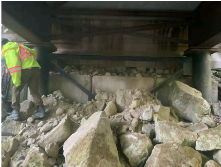
Right Bank Abutment when facing downstream
