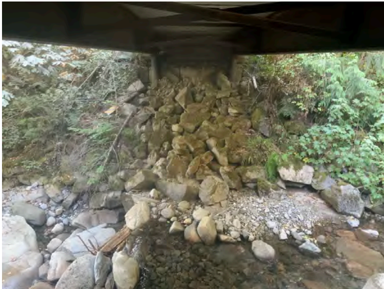
Right Bank Abutment when facing downstream
