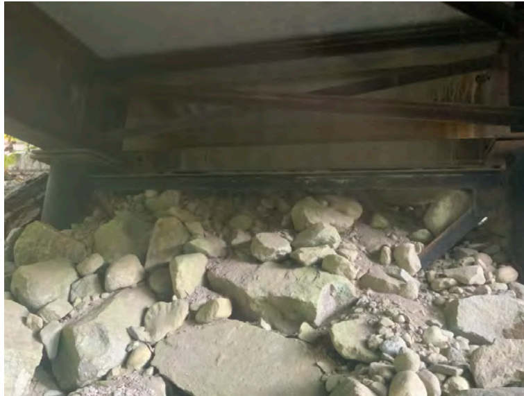
Left Bank Abutment when facing downstream
